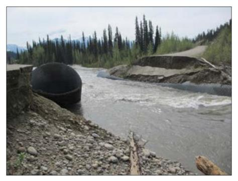
Figure 1. Washed out culvert on the Nahanni Range Road #1 (June 2012).
