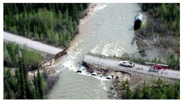
*Figure 6.* The Nahanni Range Road, which leads to the mine, was washed out in three locations; however, the culverts displayed no obvious corrosion or deformation (Yukon Department of Highways and Public Works).
