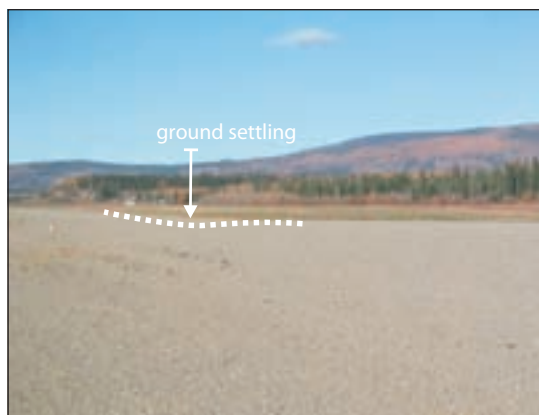
Figure 33. Examples of degradation observed on the Mayo airport landing strip.
