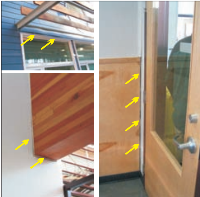
Figure 25. Examples of infrastructure damage due to permafrost thawing and ground subsidence observed at the Yukon College annex, J.V. Clark School, Mayo.
