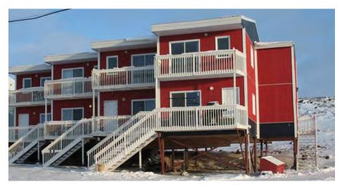
Figure F14. Example a steel-pile foundation in Nunavik (Gravel, 2012).
