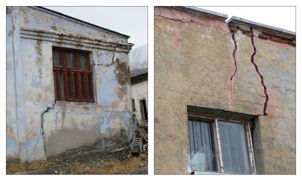
*Figure F3.* Examples of unmaintained buildings in Pyramiden, Svalbard, displaying cracks and uneven settlement in response to permafrost thaw.
