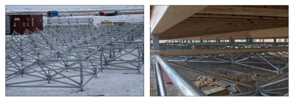
Figure F13. Examples of space-frame foundations in Nunavut (Barriault, 2012).
