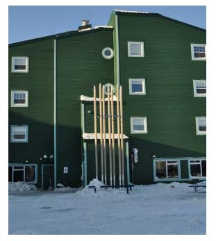
*Figure F16.* Example of thermosyphons, a foundation system that requires a significant amount of expertise to design, install, maintain and monitor (CSA, 2014).
