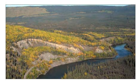
**Figure 21.** Rotational slump near km 9 of the North Canol Road (station 13DT37). Road construction and river erosion are undercutting the toe of the slide and contributing to instability. The slump is approximately 70 m tall, 250 m wide, and 180 m long.
