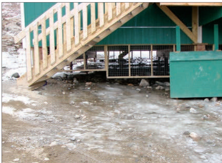
Figure C18. Example of water ponding around a foundation built on permafrost (Government of Nunavut, 2013). Water ponding can have a negative impact on permafrost thermal regimes.
