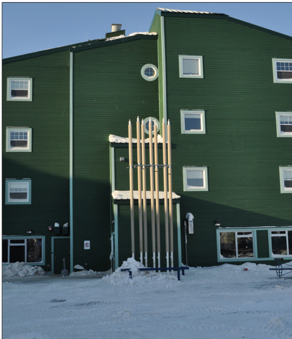
Figure C16. Example of thermosyphons, a foundation system that requires a significant amount of expertise to design, install, maintain and monitor (CSA, 2014).
