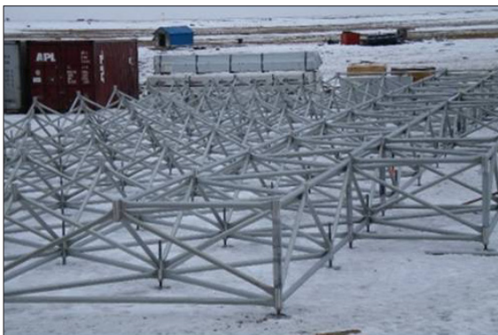
Figure C13. Examples of space-frame foundations in Nunavut (Barriault, 2012).
