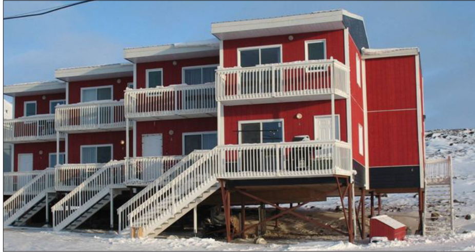
Figure C14. Example a steel-pile foundation in Nunavik (Gravel, 2012).
