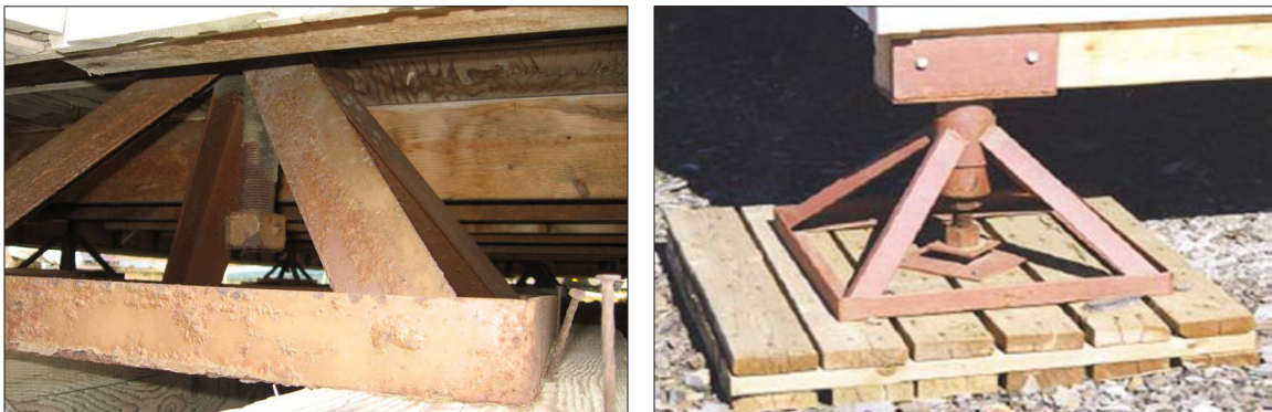
Figure C11. Examples of adjustable-jack foundations from Gravel (2012) and CSA (2010).
