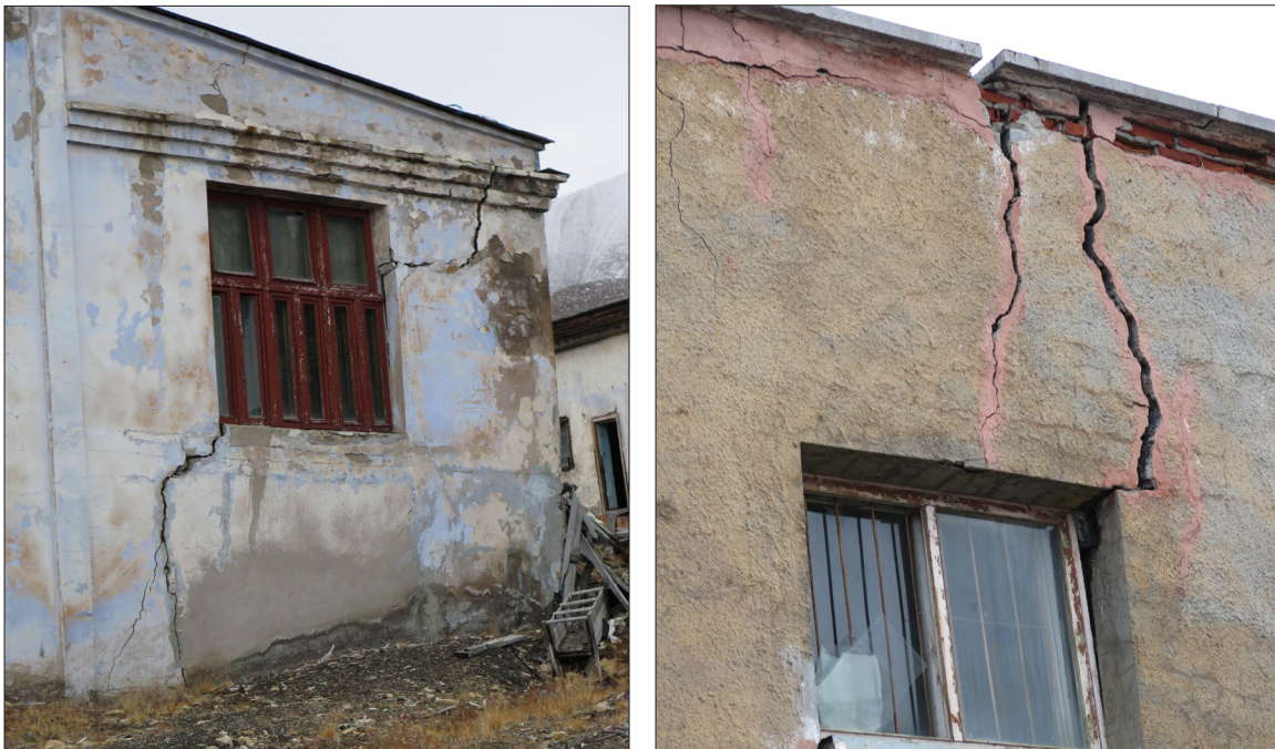
Figure C3. Examples of unmaintained buildings in Pyramiden, Svalbard, displaying cracks and uneven settlement in response to permafrost thaw.
