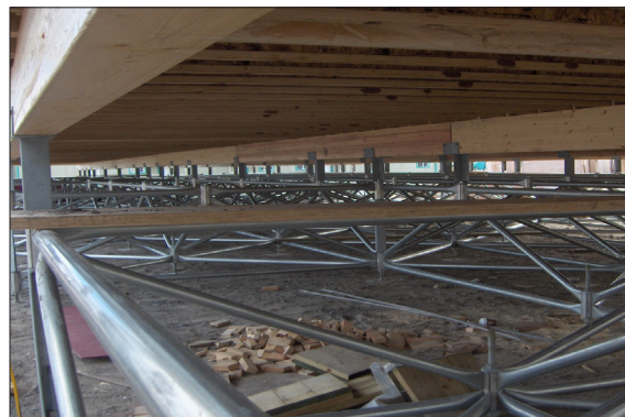
Figure C13. Examples of space-frame foundations in Nunavut (Barriault, 2012).
