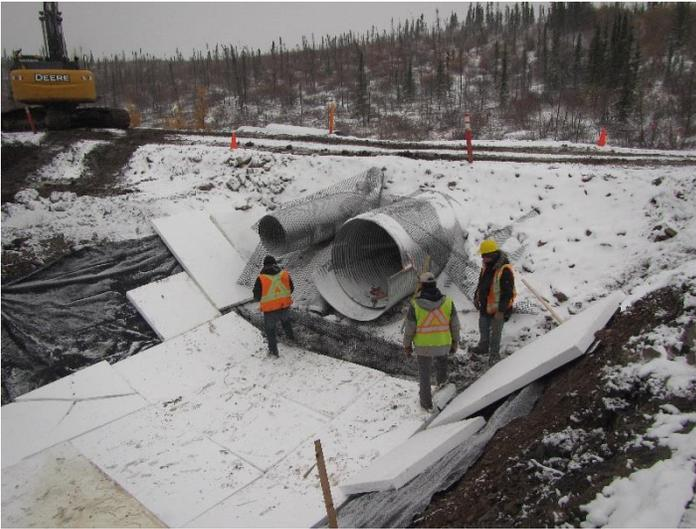
Figure 3.11 Construction of the culvert at right-hand side of the road. Note the secondary culvert located left of the main culvert. As there was an insufficient supply of foam, some areas remained uninsulated at both sides of the culvert.
