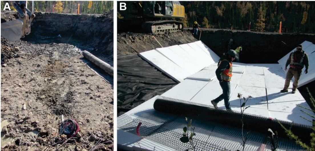
**Figure 3.9 Construction of the culvert and installation of the first monitoring array. A- excavation in natural ground; B- installation of the insulating foam.**
