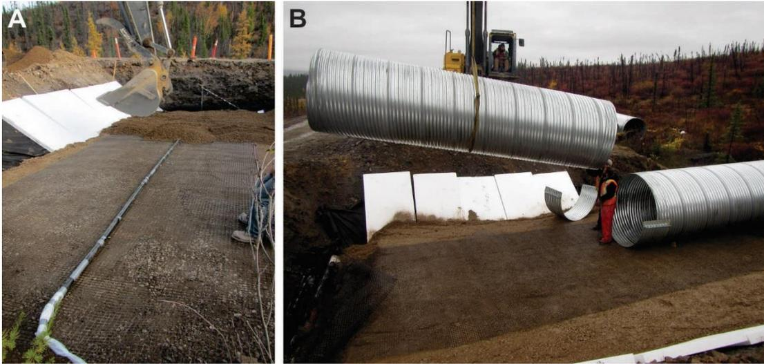
**Figure 3.10 Construction of the culvert and installation of the second monitoring array. A- excavation in natural ground; B- installation of the insulating foam.**
