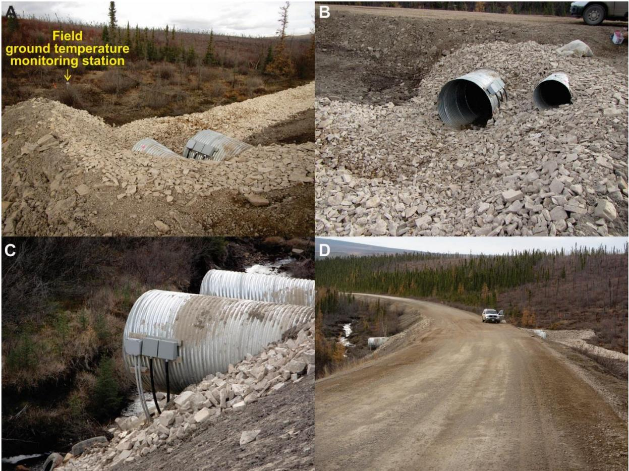
**Figure 3.15 Culvert site at km 381 after construction. A- view from the road on the left-hand side showing the station monitoring the natural ground temperature in the field; B- view from the field showing the left-hand side of the embankment; C- view from the road of the right-hand side; D- general view of the site from up-slope.**
