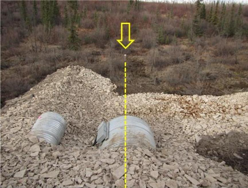
**Figure 3.14 Borehole DH381 BH1, located in the field, right-hand side, aligned with the center of the culvert and the buried monitoring array lines (location of the station indicated by the yellow arrow).**
